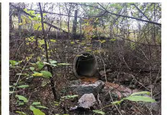
Outfall pipe of tributary that runs beneath path.
