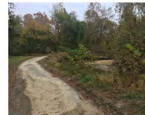
The asphalt path lies within feet of the stream bank.
